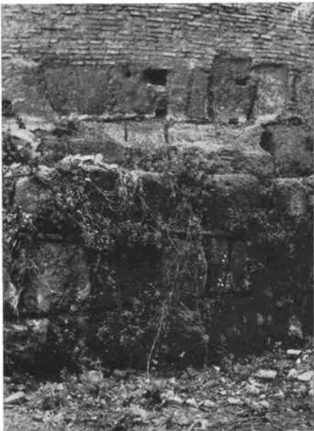
Fig. 96d. S. Martino ai Monti, Ninth century basilica, foundation wall and platform of apse
